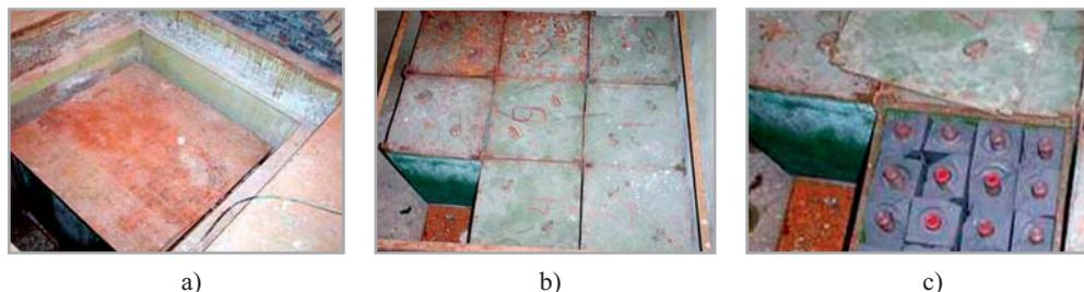
**Figure 5.** The frame with the containers in the pit (a), eight containers with fuel blocks (b), fuel blocks in one of the uncovered containers (c)
