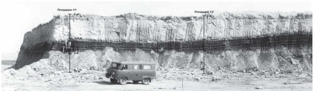
**Figure 6.** General view of Block A fragment before mining (dark-color stratum is the rock with elevated NRD concentration)
