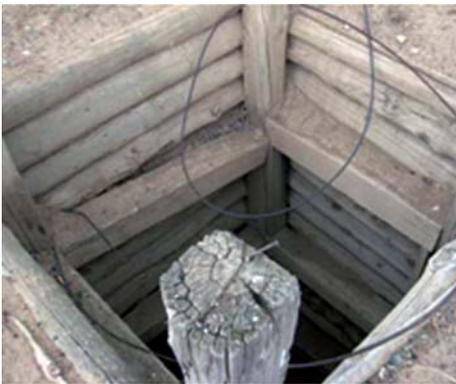
*A wooden construction like a well, depth 5 m*
