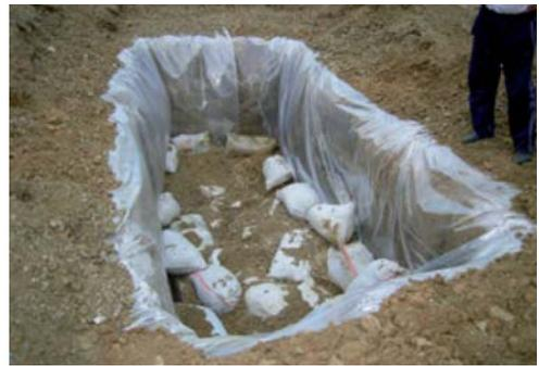
**Figure 30.** Disposing of radioactive scrap metal and soil in MPTO-10
