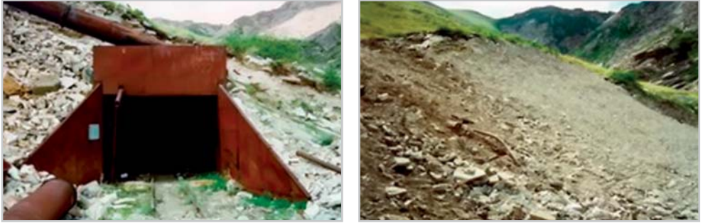
Figure 33. Entry to the tunnel №022 before and after closing
