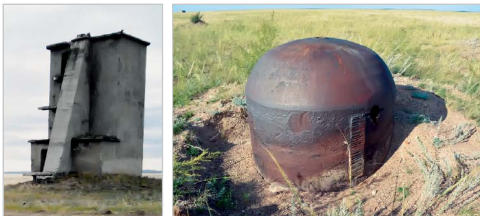
Figure 20. Strong 4-storeyed reinforced concrete instrument structure of “goose” stiffening rib. Located at the P-1 technical site. Armored hood in a permanent fire position (PFP) is to the right
